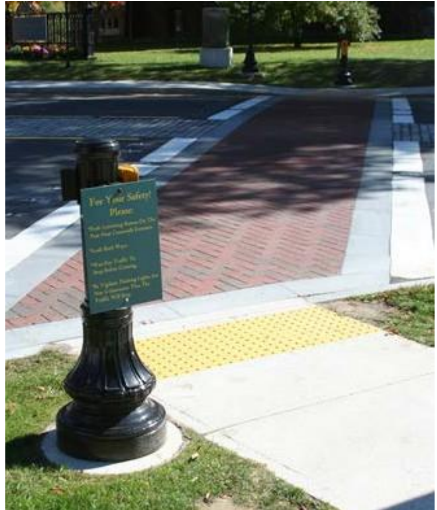
Wide cross walks, clearly marked and built with durable, high quality and attractive materials enhances the safety as well as the character of town centers. Cross walk lights that reduce pedestrian waiting times to less than a minute and a half are also desirable.
