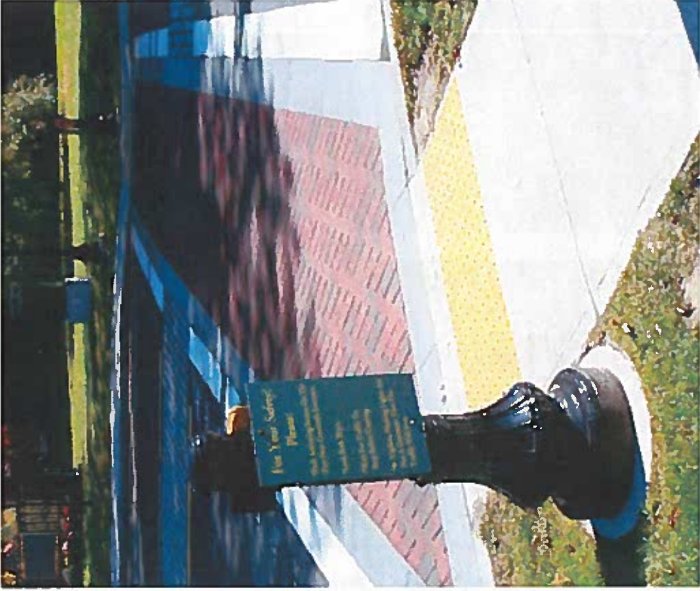
Wide, accessible cross walks, clearly marked and built with durable, high quality and attractive materials enhances the safety as well as the character of town centers. Cross walk lights that reduce pedestrian waiting times to less than a minute and a half are also desirable.
