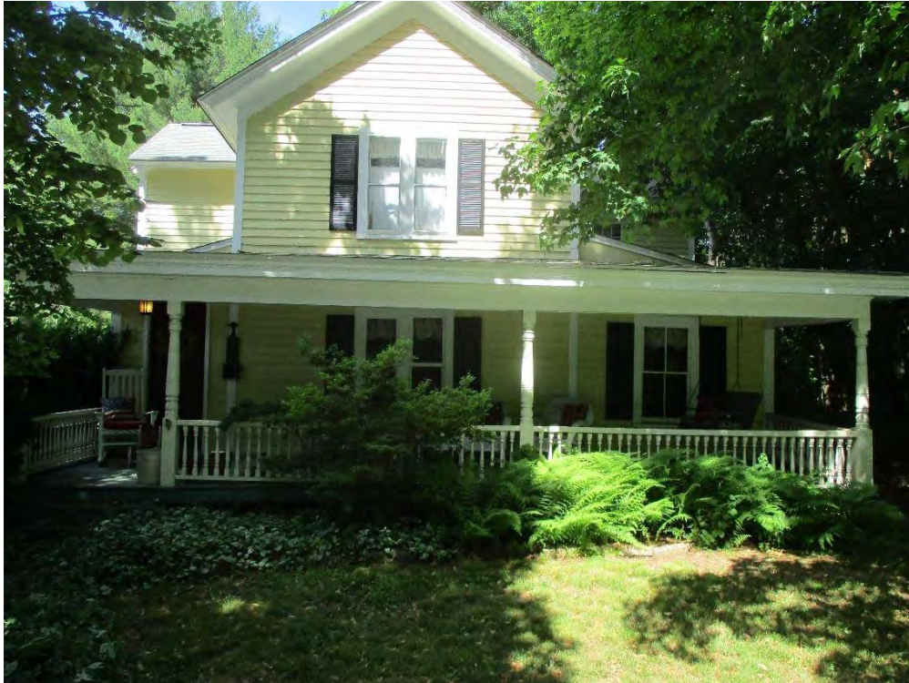
Asa Hawley House, 796 Plainville Avenue, built ca. 1800. East elevation.
