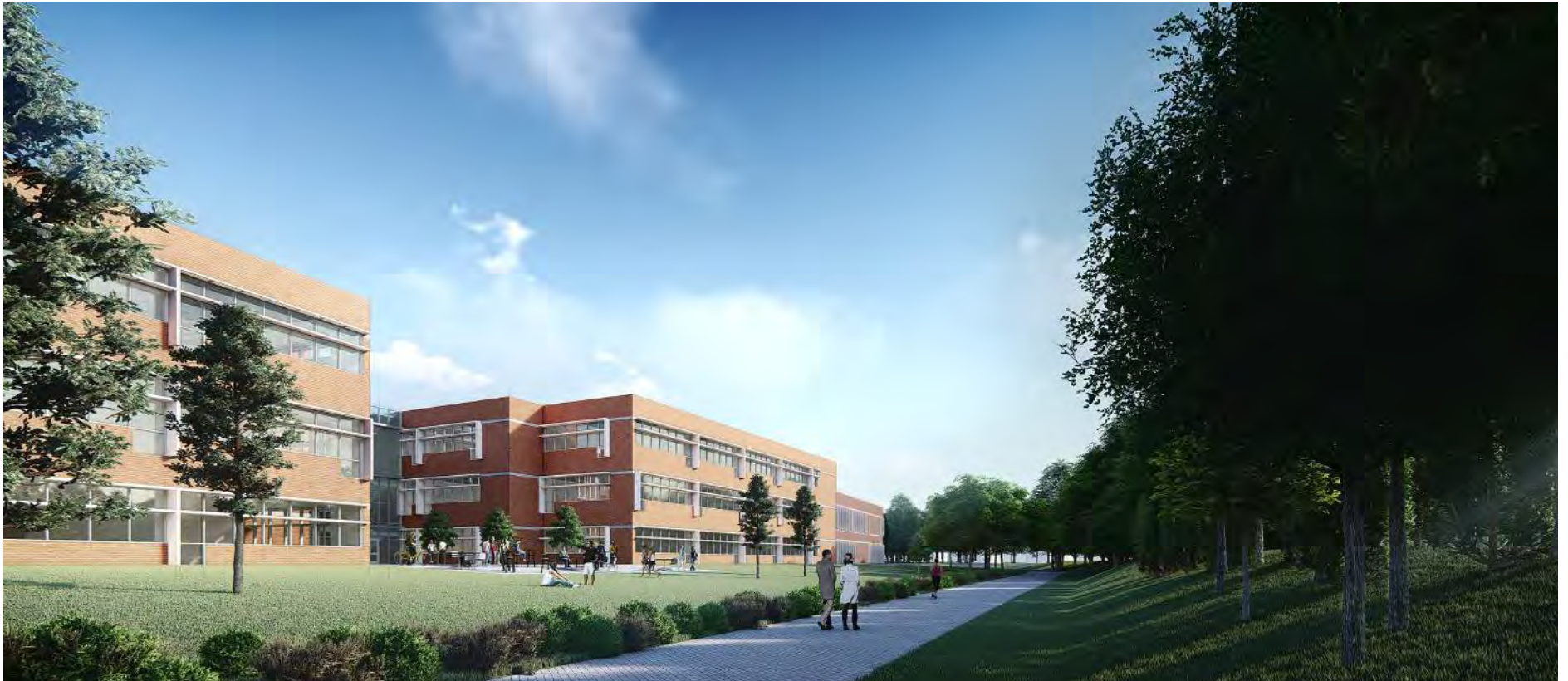
View along eastern edge of property
