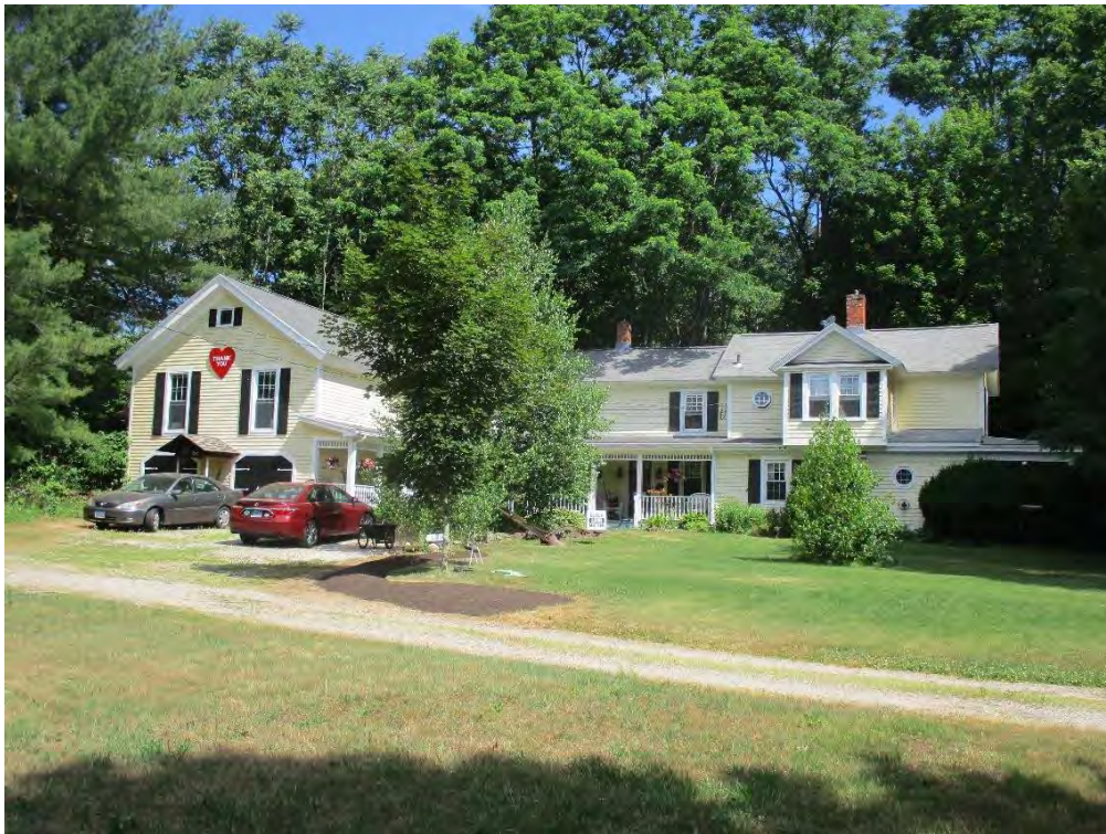
Asa Hawley House, 796 Plainville Avenue, built ca. 1800. South elevation.
