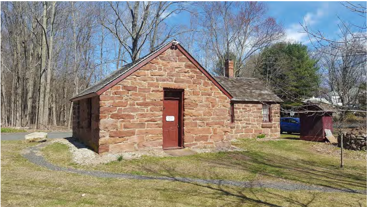
Old Stone Schoolhouse/The Chapel, 93 Coppermine Road, Farmington CT
