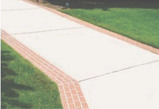
WIDER SIDEWALK TREATMENT WITHIN LAWN AREA
