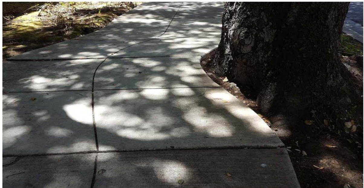
Figure 11. City curved the sidewalk around the mature oak's trunk to provide extra space (Palo Alto).
