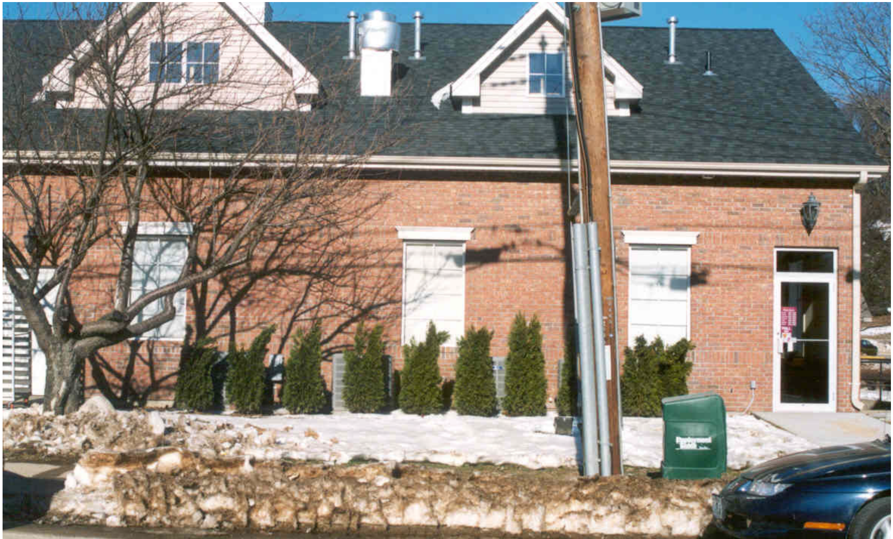
This Dunkin' Donuts has screened their utilities with evergreen Arborvitae. When these plants reach maturity the building's utilities will not be visible from the street.
