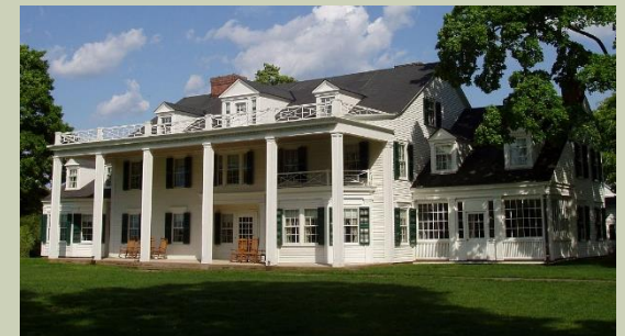
2 ½ Story 110 Foot Long West Façade
