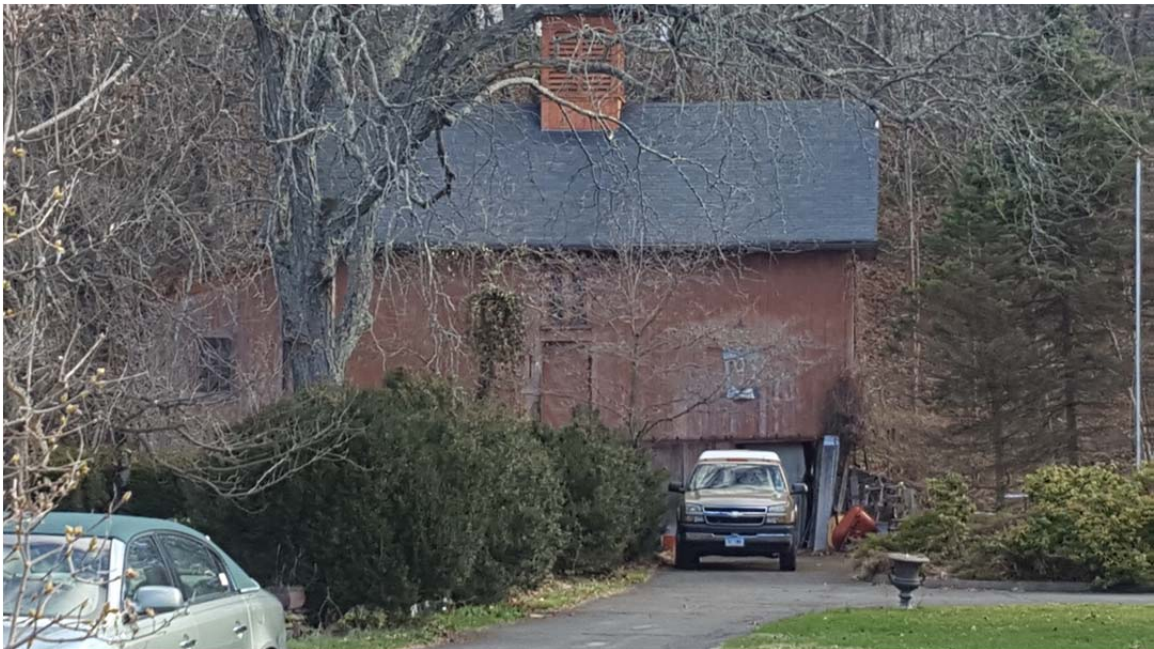
Bank barn, 230 Main Street, Unionville
