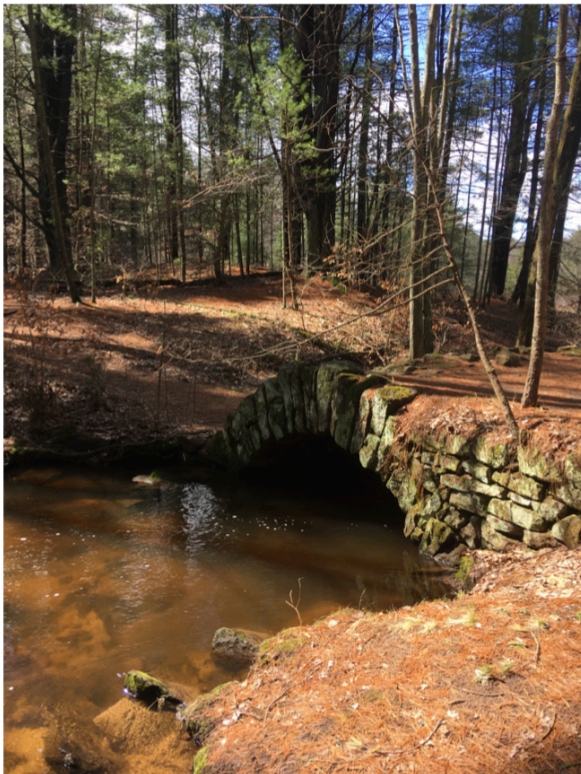
Thompson Brook Culvert
